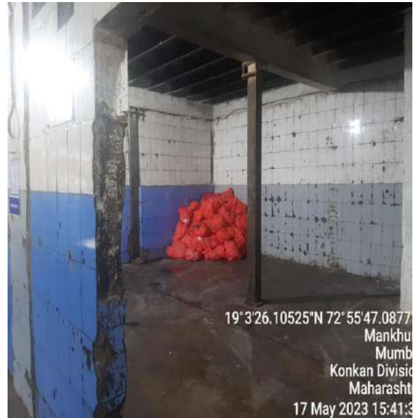
Photograph-6: Designated colour coded BMW storage room for red category of BMW.
