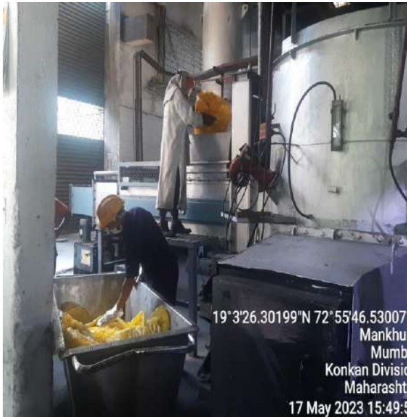
Photograph-9: Feeding yellow category BMW into the incinerator and the personnel engaged not wearing adequate PPE i.e. hand glove and wearing ordinary mask.
