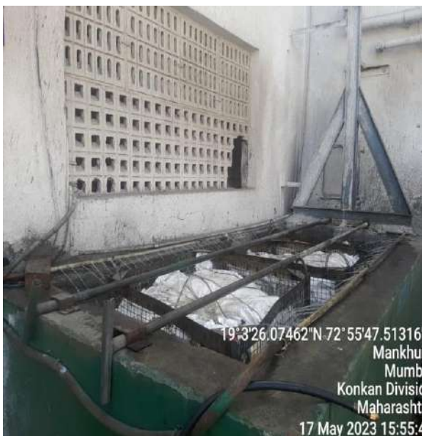
Photograph-11: Treatment of blue category BMW with disinfection.
